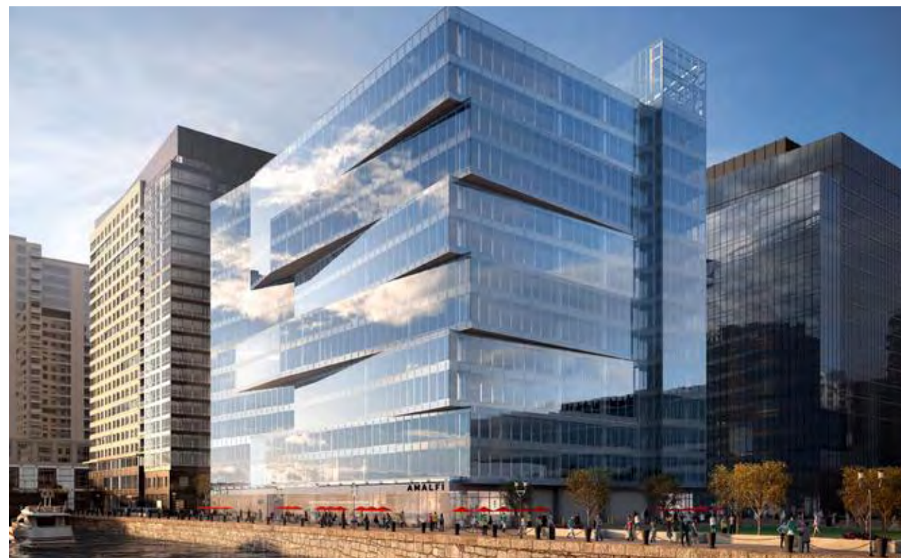
Pier 4 — Boston, MA
